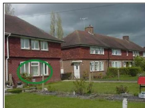
Post War property where plastic double glazing, with no trickle vents, has been added and can cause condensation.
