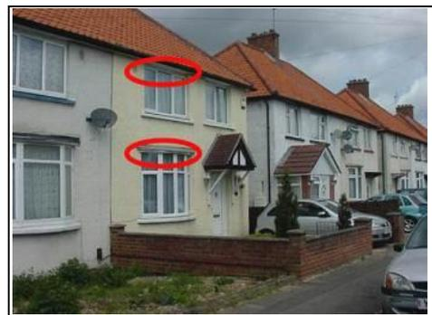
Thermal and cold bridging can be caused in War Years properties by cold elements in the structure such as lintels over windows and doors
