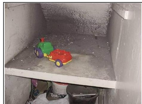
Black mould in cupboard due to lack of air circulation
