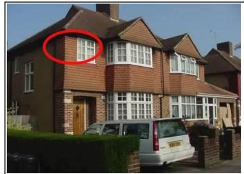
1930s properties can be more susceptible to thermal and cold bridging where rooms are formed partly in the roof
