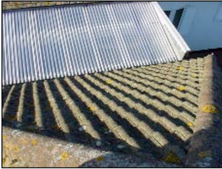
A view of the right hand side of the hipped roof
