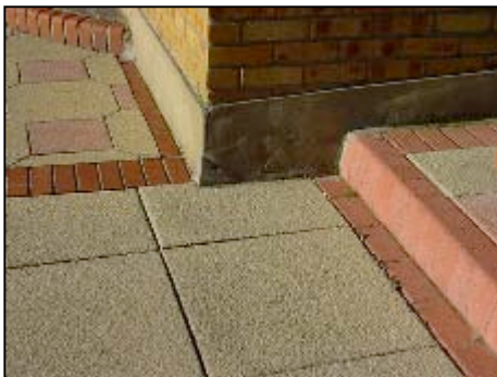
Render to the base of the brickwork
