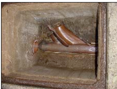
Manhole finished in concrete.
