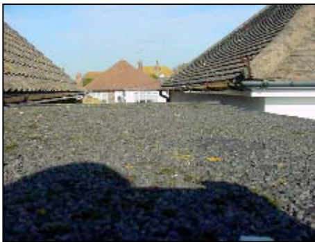
An older style flat roof
