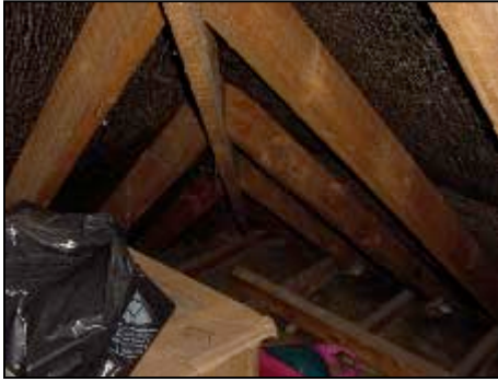
A view of the corner of the roof, which is an area where hipped roofs normally slip, as you can see in this instance there is no problems.
