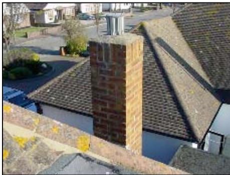
Left hand brick chimney
