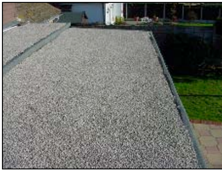
A view of the rear low-level flat roof.
