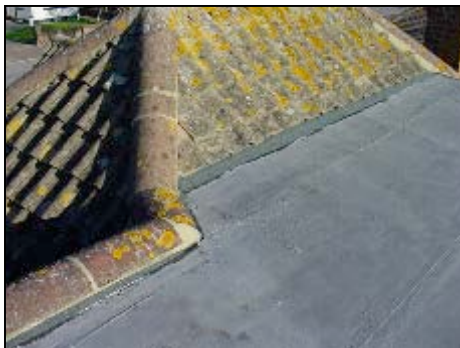
A view of the high level roof
