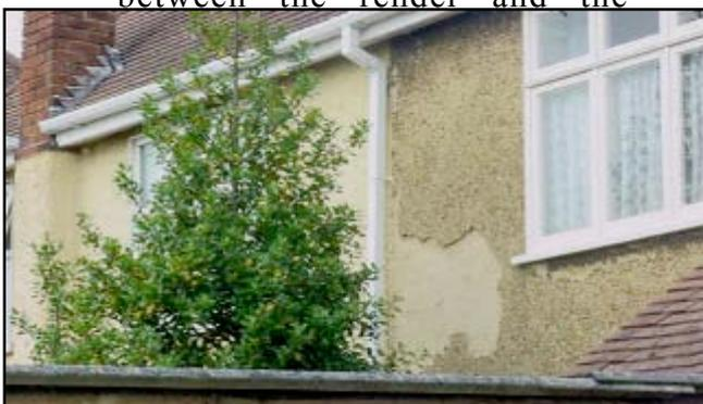
To the right hand side of the bush you can see the render deteriorating. This can start to occur where **Time** cracks are found within the
