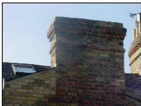
Rear chimney in reasonable order.
