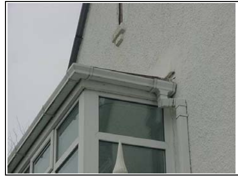
Close up of the Bay Window Roof
