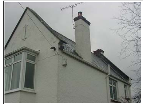
Close up of the Flashing
