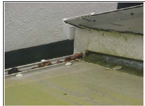
Leaves in a low level gutter
