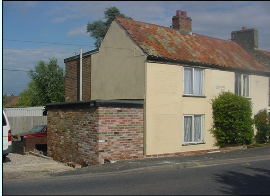
The finished brickwork
