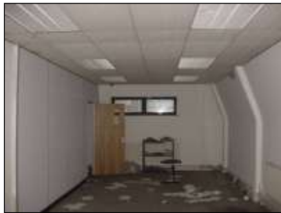
Office and Kitchenette
