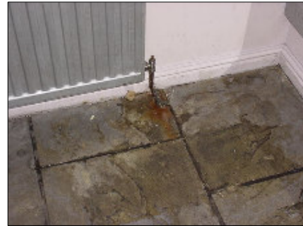
Leaking radiator and ingrained dirt to flagstones
