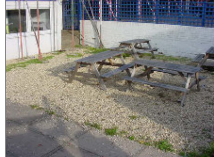
Weeding required to shingle part of patio area
