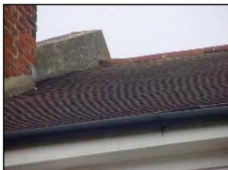
This shows how flat the concrete tiles sit on the roof, which indicates to me that they have been machine made. Also to the rear you can see the chimney and the render covered parapet wall together with some ridge tiles.
